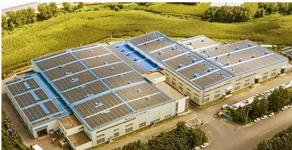
Photovoltaic panels installed on the roof of our Shenyang, China, plant.
